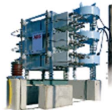
Filter capacitor installation
