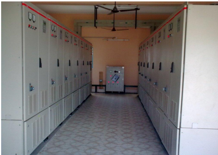
Figure 20 : Typical Railway STATCON + MV Capacitor Bank Installation
