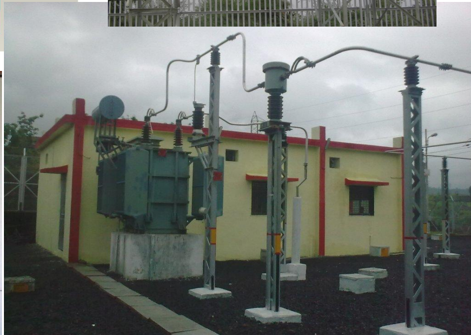
Figure 20 : Typical Railway STATCON + MV Capacitor Bank Installation
